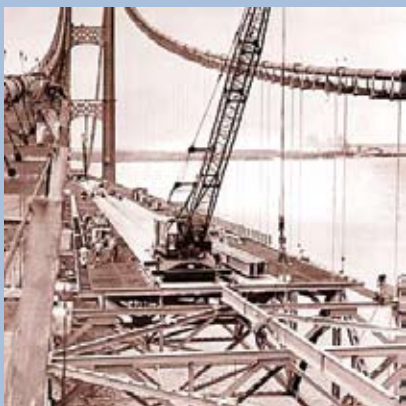
Building the Mighty Mac 50th Anniversary Addition
